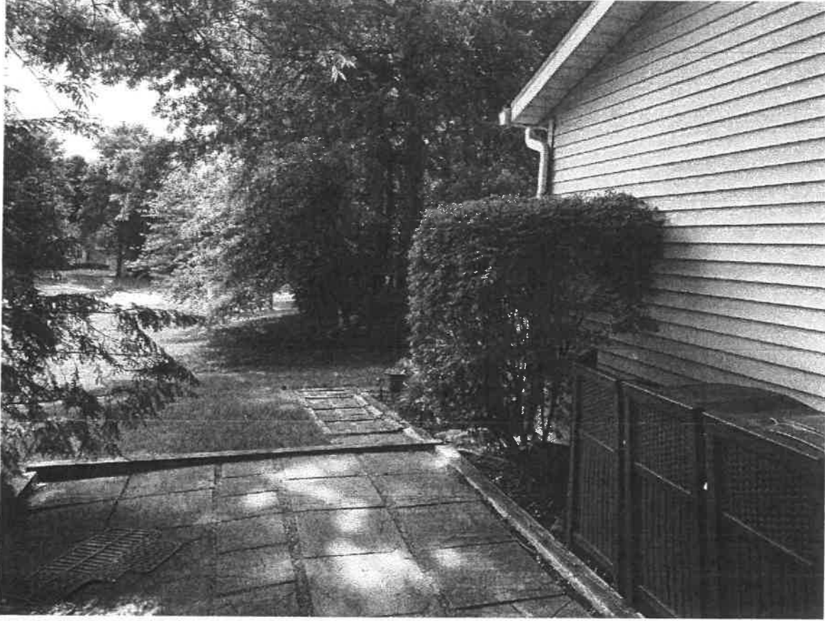
8786 SMOKERISE DRIVE – VIEWS OF SOUTHWEST CORNER OF THE HOUSE
