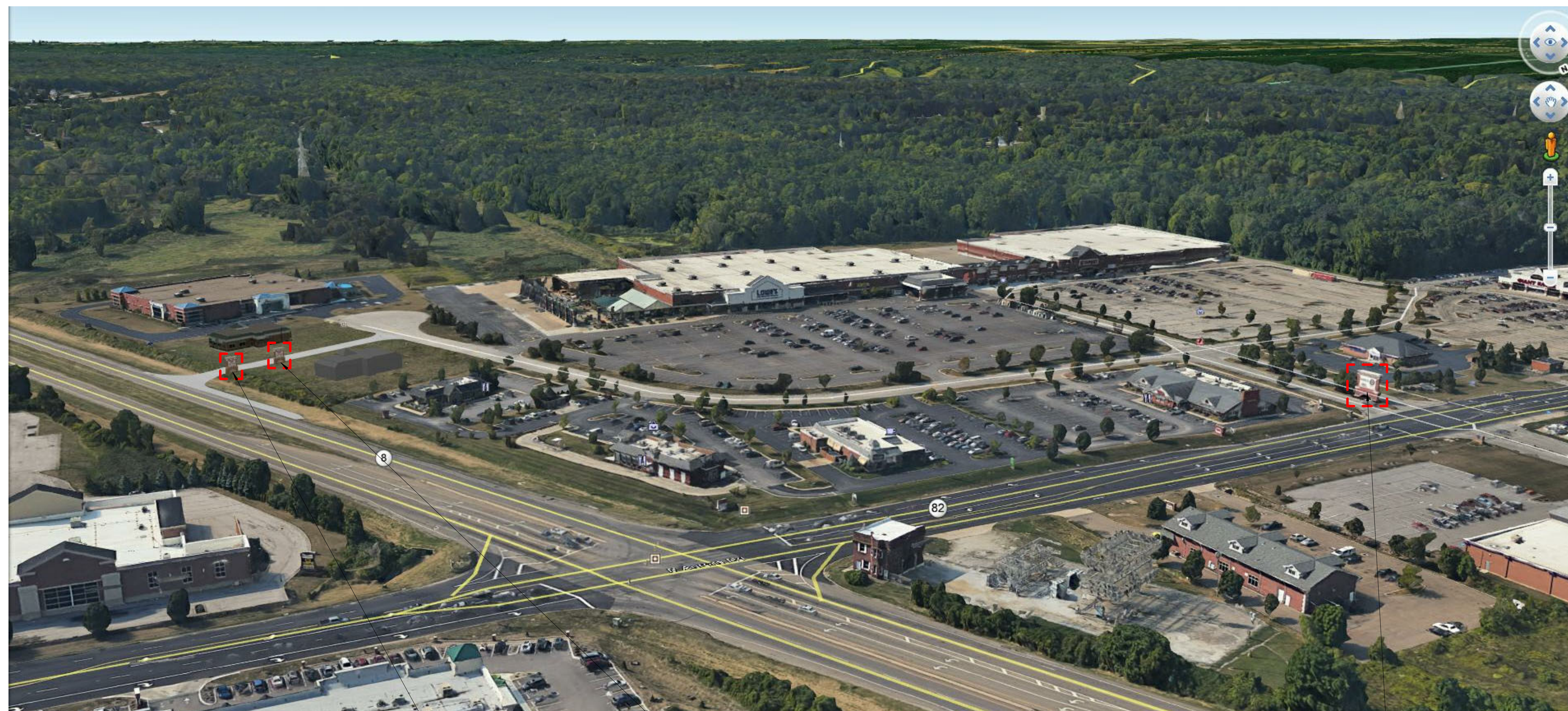
NORTH AERIAL VIEW INTERSECTION OF OH-8 AND E AURORA RD
