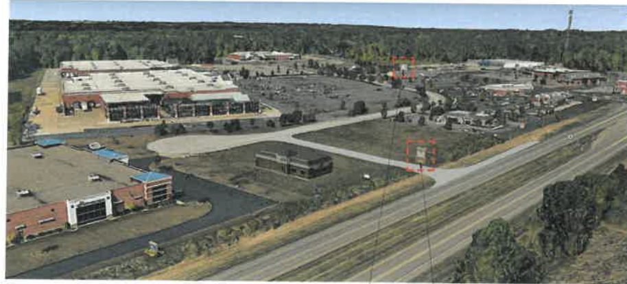
SOUTHEAST AERIAL VIEW OH-8
