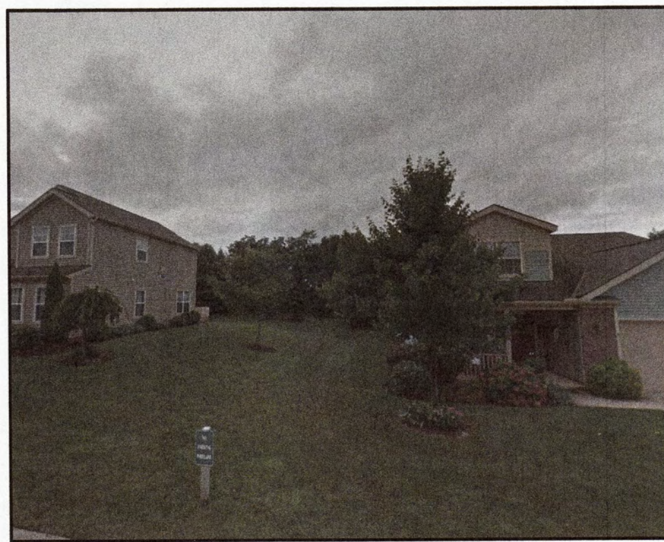
DENSE EXISTING EVERGREEN SCREENING HEAVILY RESTRICTS ANY VISUAL IMPACT
