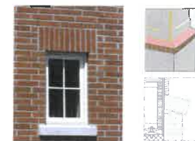
BRICK: Soldier Course and Rowlock Example and Detail
