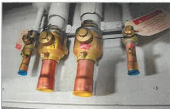
◀ Labeled split system piping stub outs with shut-off valves allow for easy installation.
