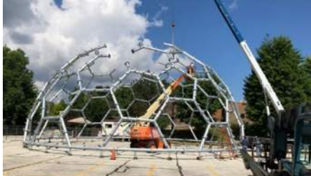
RainForest Dome Replacement Cleveland Metroparks Zoo | Cleveland, OH
