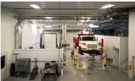
Orange Village Service Center Orange Village, OH
